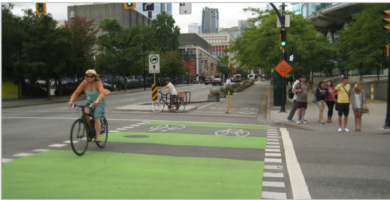
“Green pavement markings used to highlight motorist/bicyclist points of conflict in the roadway.” (2014 IL DOT Plan, p. 22)
