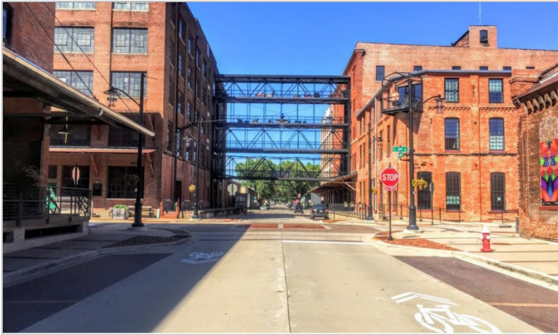
Curb extensions/ bump-outs shorten the crosswalks in the Historic Millwork District (2107 Imagine Dubuque Plan, p. 5-16)
