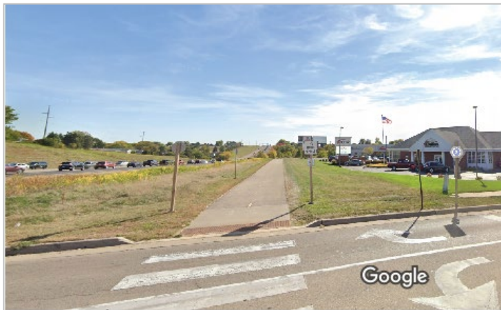
Northwest Arterial Trail (Source: ECIA using Google Maps)
